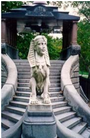
1872 Barney Mausoleum, Springfield, MA. Structural engineering restoration by CBI Consulting, Boston, MA (photo courtesy of CBI Consulting)
