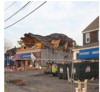
Danversport Bakery and Danversport Pizza Factory at the corner of Bates and Water Streets destroyed in November 22, 2006 explosion in Danvers, Massachusetts. (photo courtesy of Danvers Building Department)
